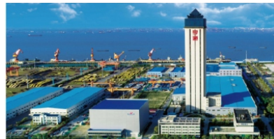
Hengtong Changshu International Marine Industrial Park
